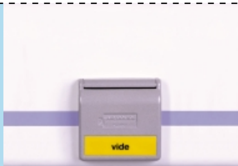
Vacuum BM terminal unit trunking mounted
